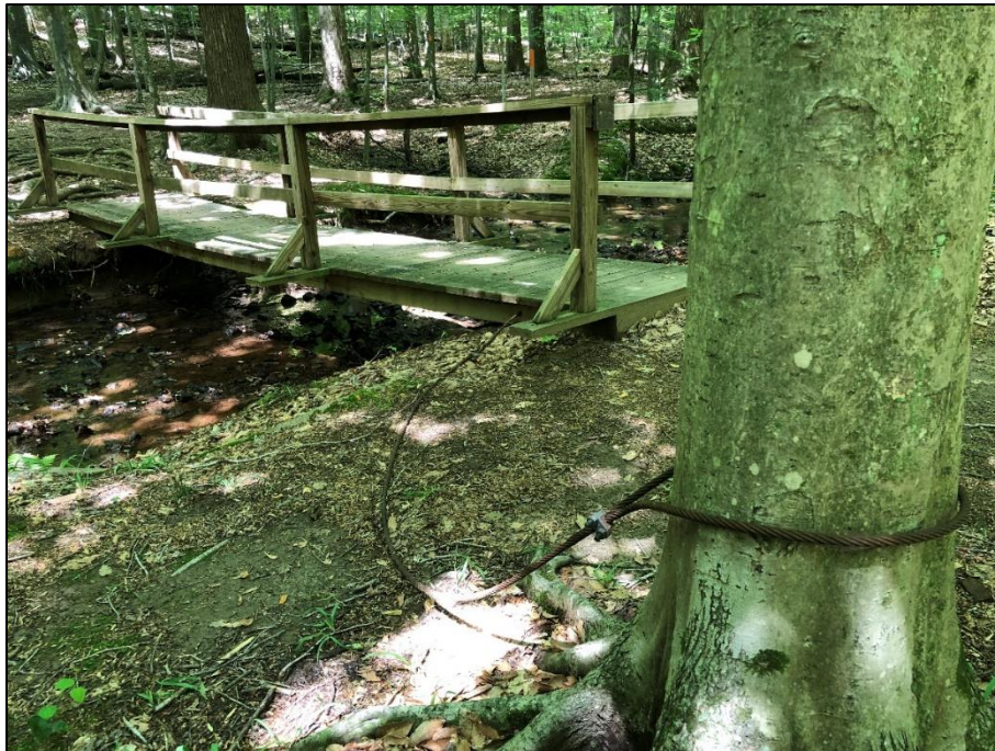
Sawn Timber Stringer Bridge with Cable, Prince William Forest Park, Triangle, VA
