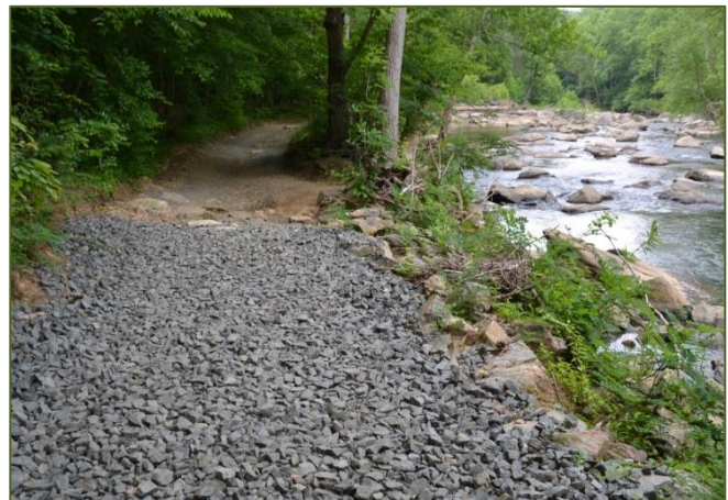
Difficult Run Trail with recent repairs of wash out due to flood event
